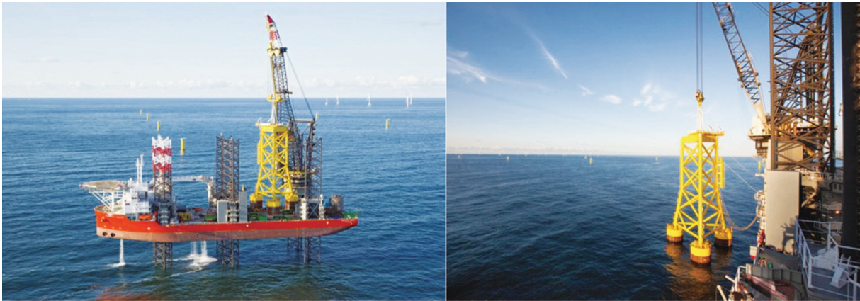
圖4 Borkum Riffgrund 1離岸風場套管式負壓沉箱基礎施工實景(Ørsted company website, 2014)
